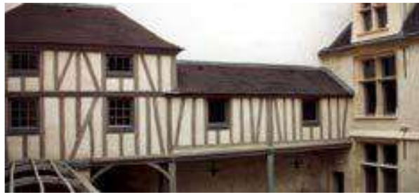
Figure 8. Restoration of 16th century historical building walls with industrial hemp
